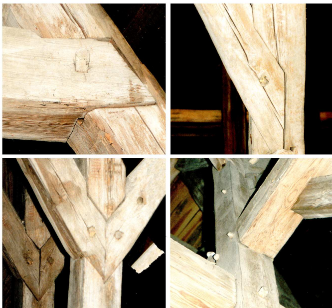
Fig. 5. Construction joints of the roof structure of the church in Grzywna/Griffen
