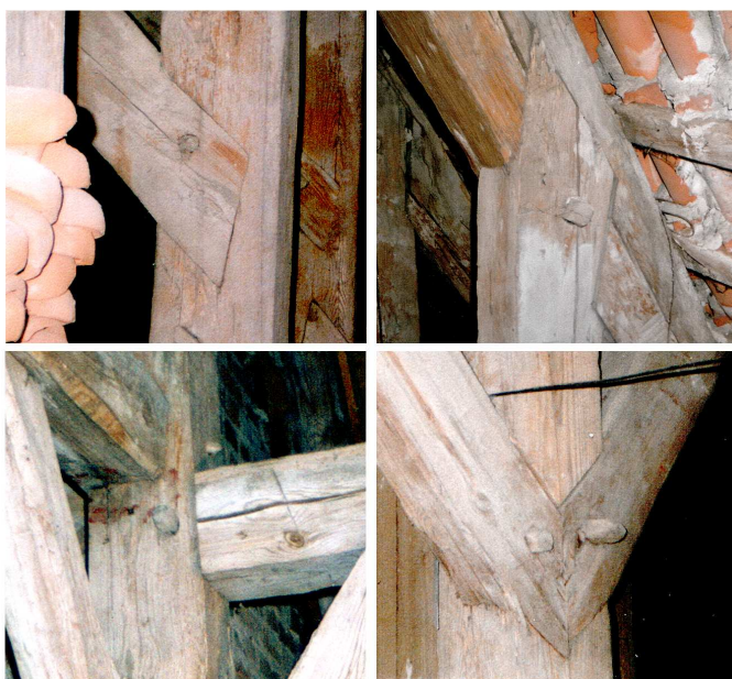
Fig. 3. Construction joints of the roof structure of the church in Lisewo/Liessau
